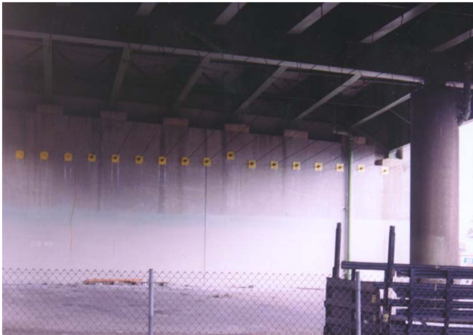
Anchor plates at Abutment
