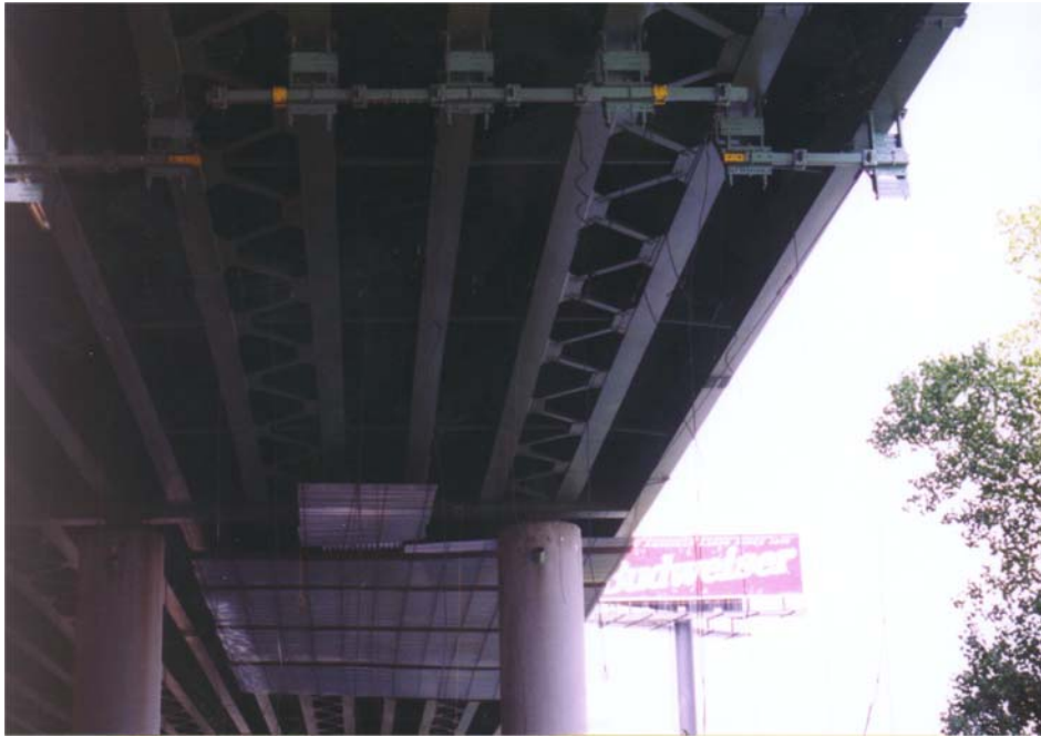
Partially installed Cable/Metal Deck Platform & Post Bracket End Connections
